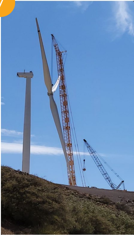
Photo 7: Hoisting turbine rotor for installation.
