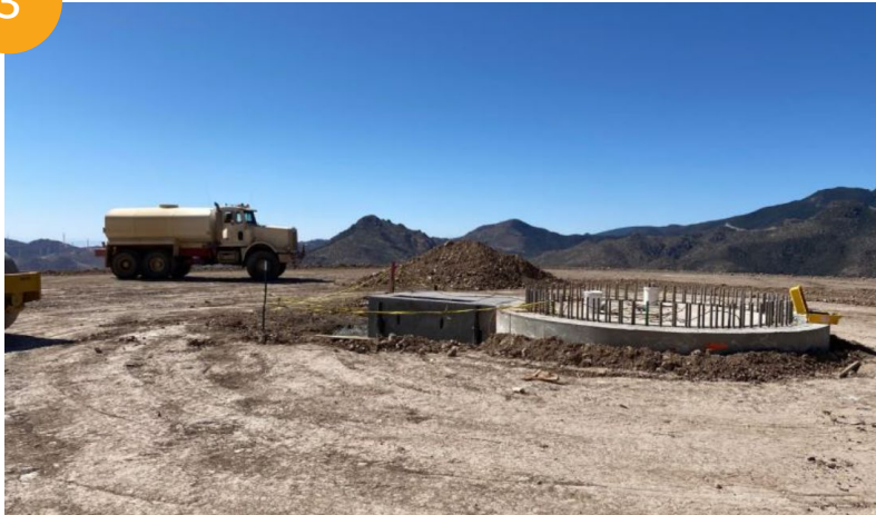
Photo 3: Concrete footing for 3 MW Siemens Gamesa turbine.
