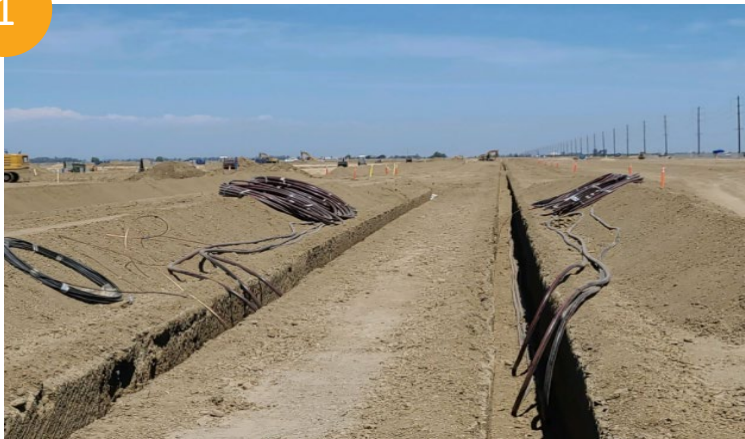
Photo 1: Onsite trenching for mid-voltage cabling.
