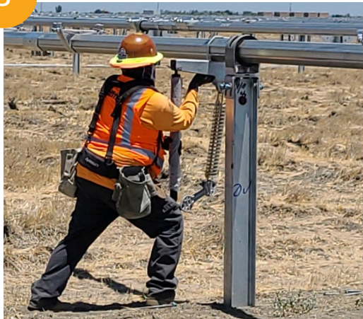
Photo 3: Racking installation with strut assembly.
