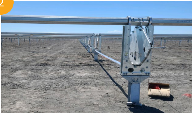
Photo 2: Tracker driveline installed to enable single-axis panel rotation to maximize solar output.
