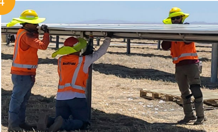
Photo 4: Photovoltaic module installation.
