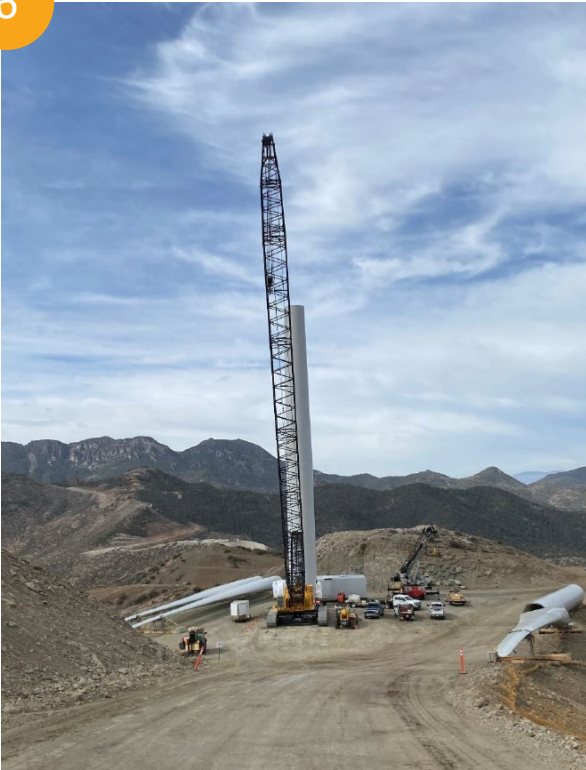
Photo 6: Installation of tower midsection.
