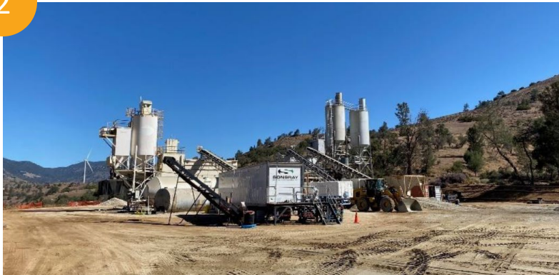
Photo 2: Assembly of concrete batch plant.
