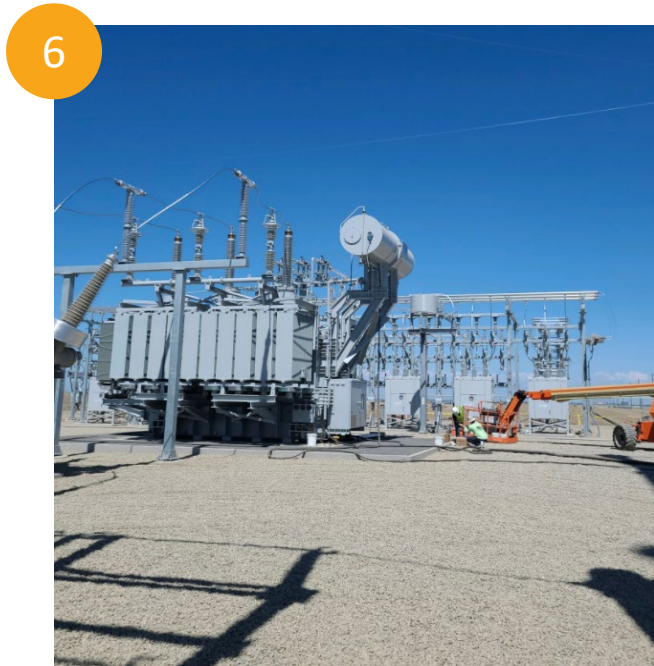
Photo 6 : Termination of gen-tie line to the project substation.
