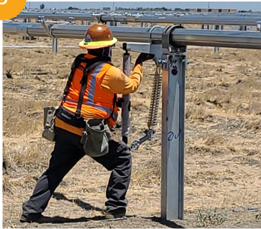
Photo 3: Racking installation with strut assembly.
