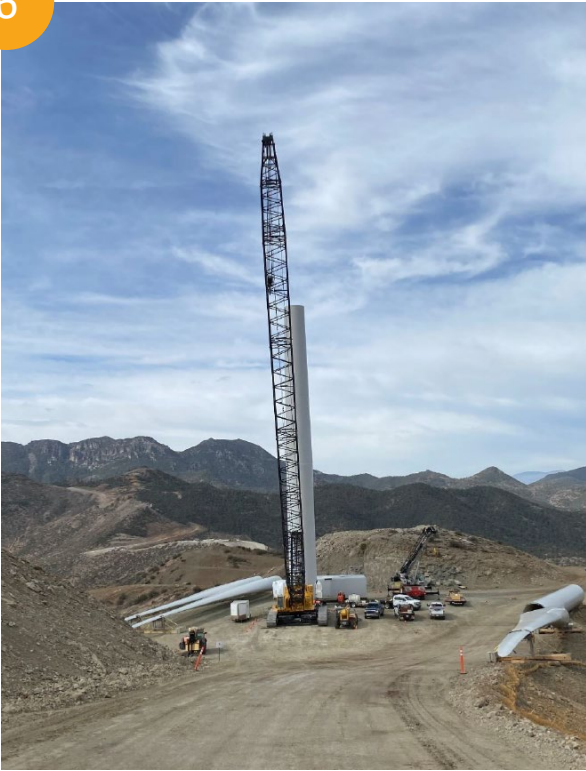
Photo 6: Installation of tower midsection.
