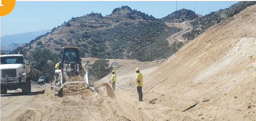
Photo 1: Onsite trenching for mid-voltage cabling.
