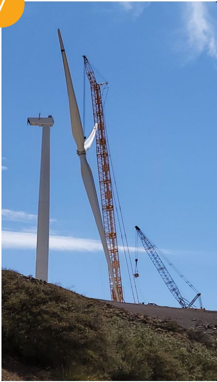
Photo 7: Hoisting turbine rotor for installation.
