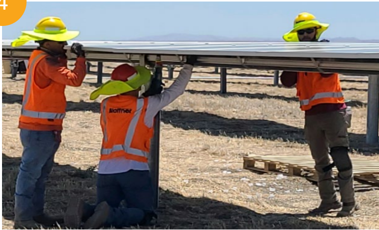
Photo 4: Photovoltaic module installation.
