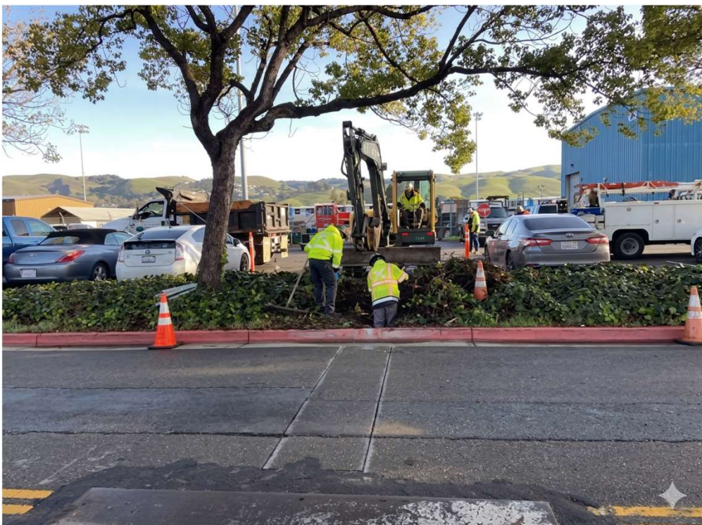
Construction Crew at the Hayward Yard
