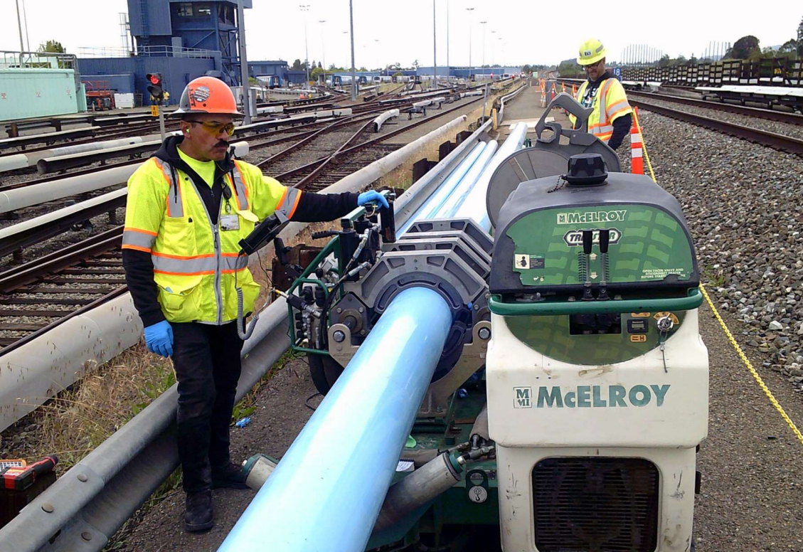
Construction Crew at the Hayward Yard
