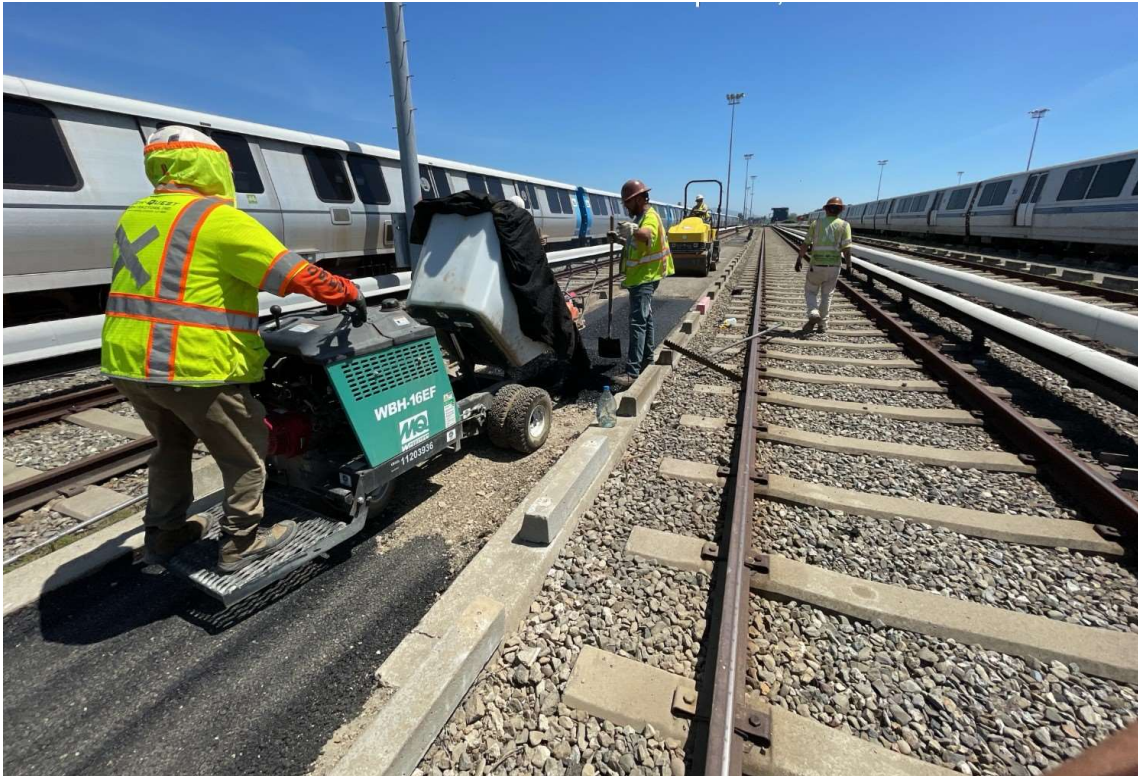
Construction Crew at the Hayward Yard
