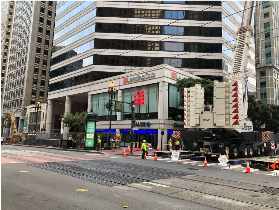
Setup for Lifting & Lowering of Substation Equipment at Montgomery Station
