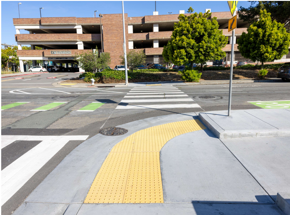
Improved Cross-walks, ramp and Bikeways near the BART Station
