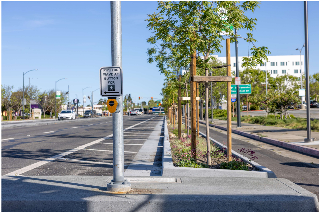
During Construction near the El Cerrito del Norte BART Station
