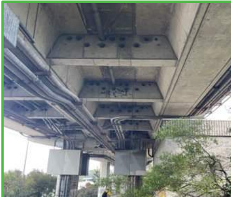
Site Survey for installing under Daly City Guideway
