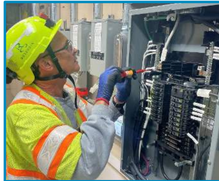
Power Panel installation at Colma
