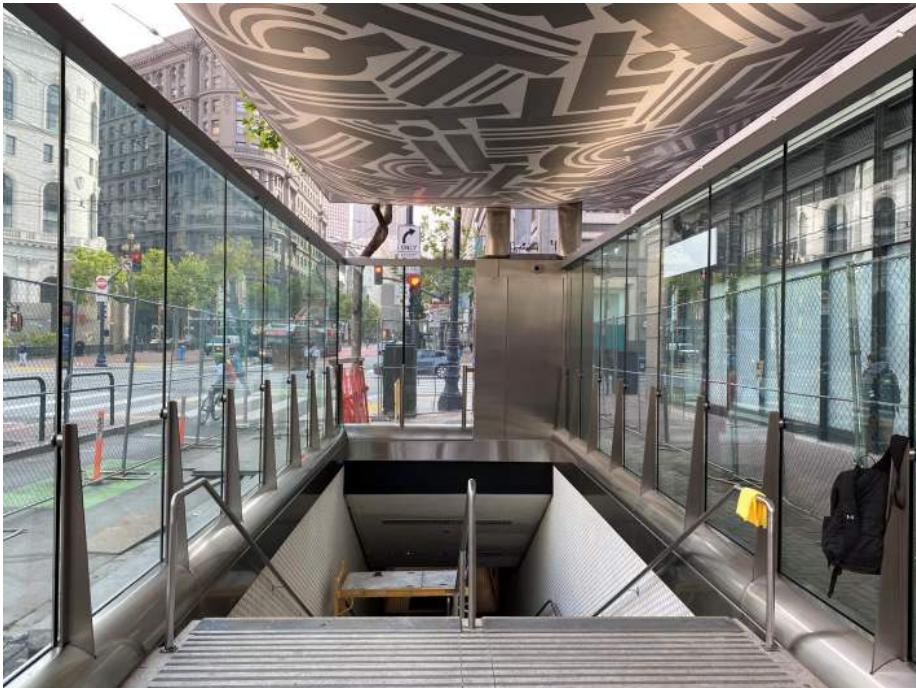
Powell Street Canopy Near Completion
