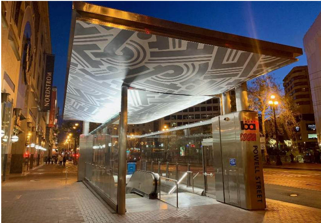
Entry Canopy at Powell Street Station
