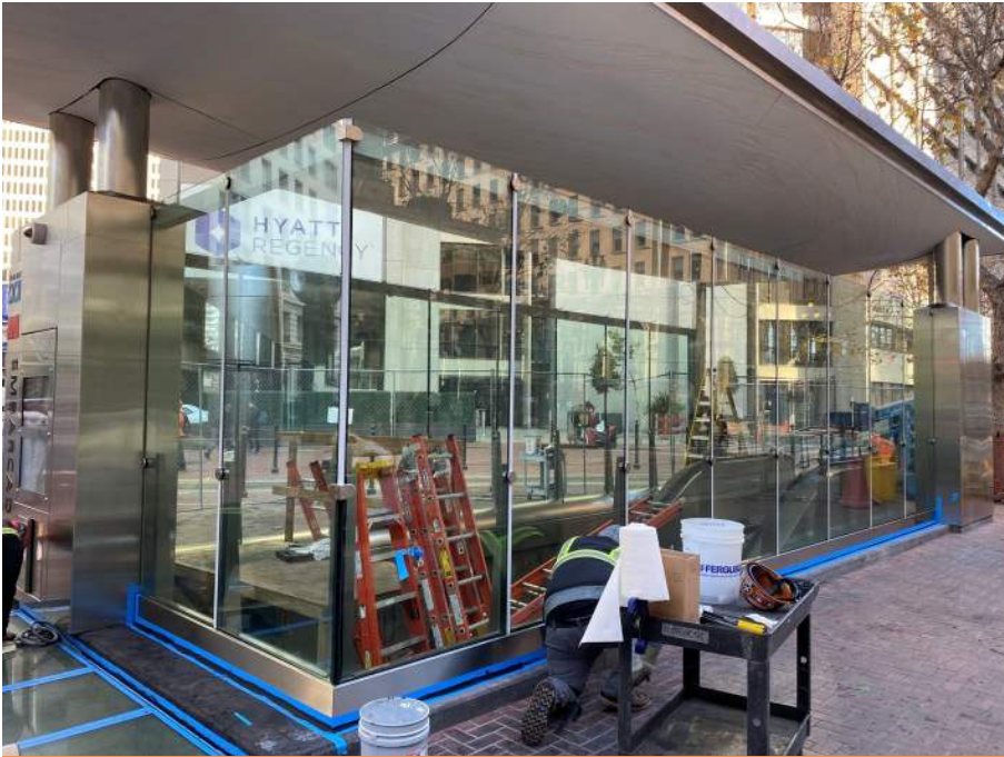
Embarcadero Canopy Under Construction
