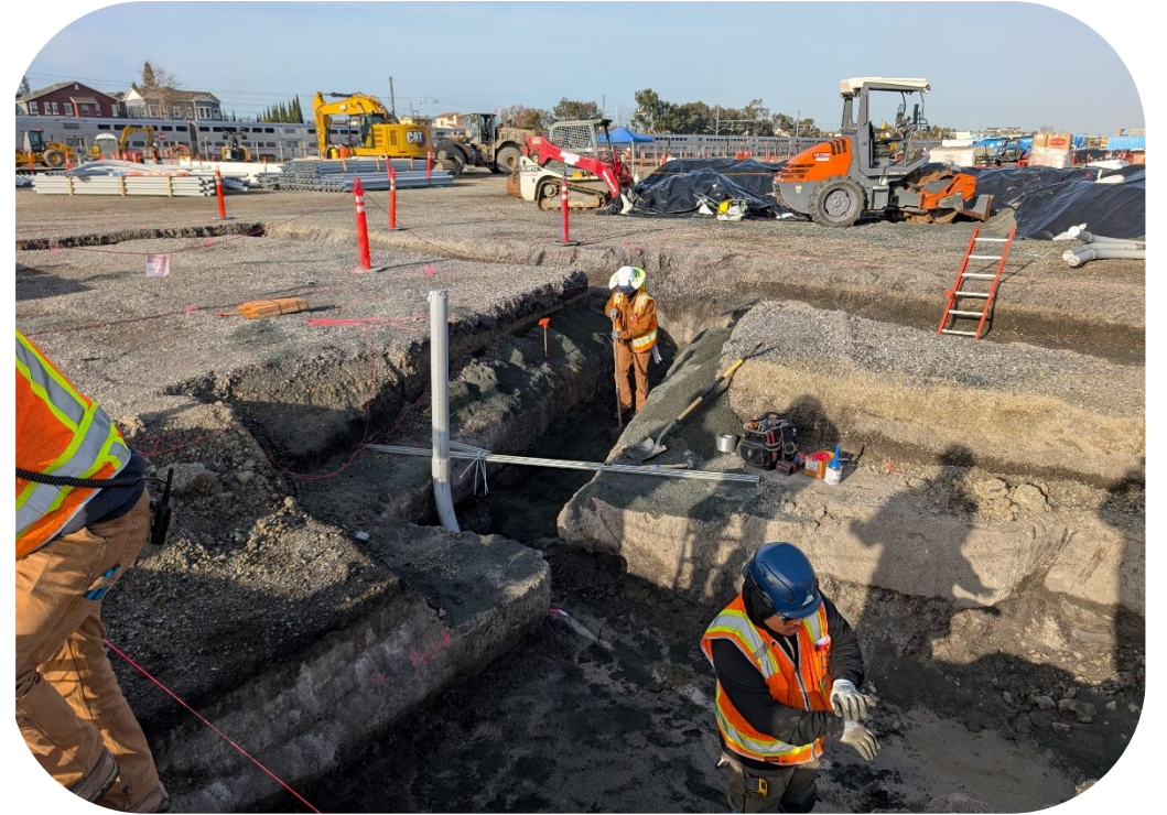
Installing lateral utility connections.
