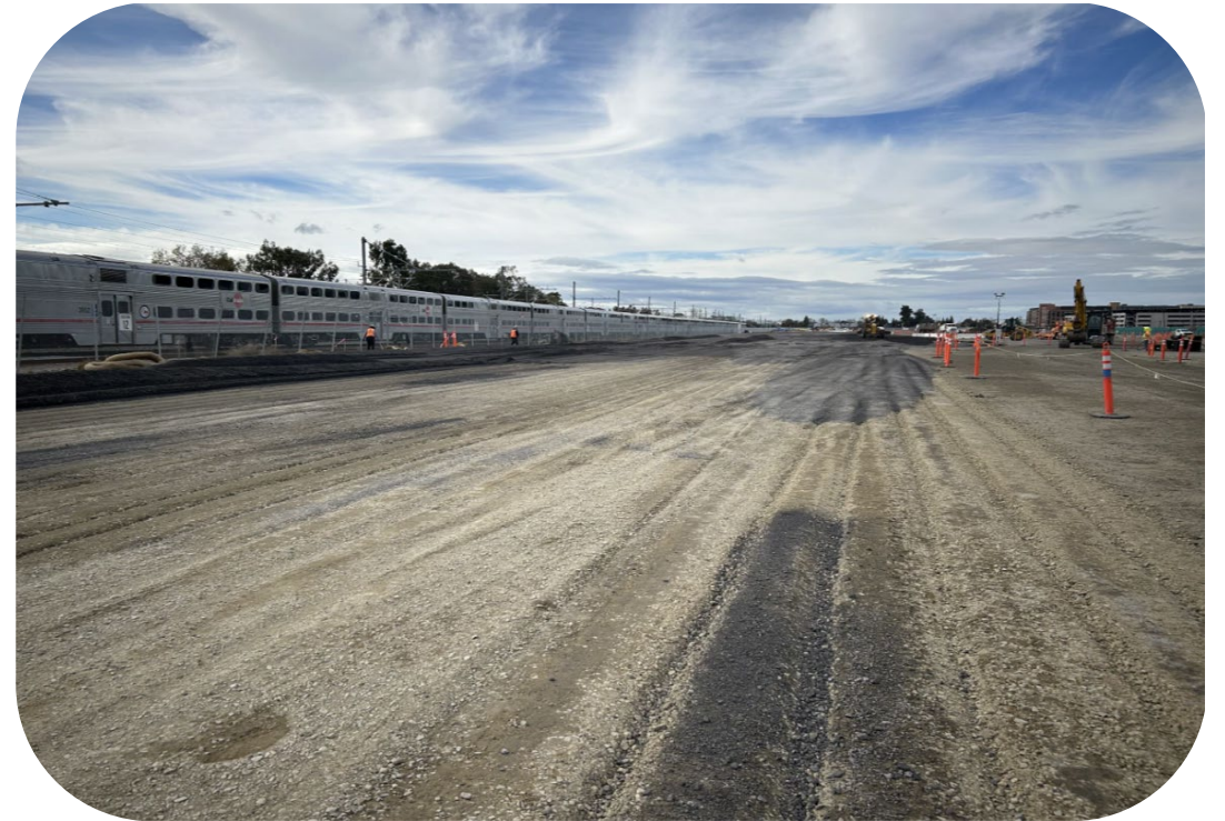
Grading complete for top of launch structure.
