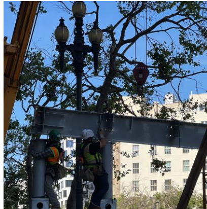
Tree Removal Tree Conflict with Entry Canopy
