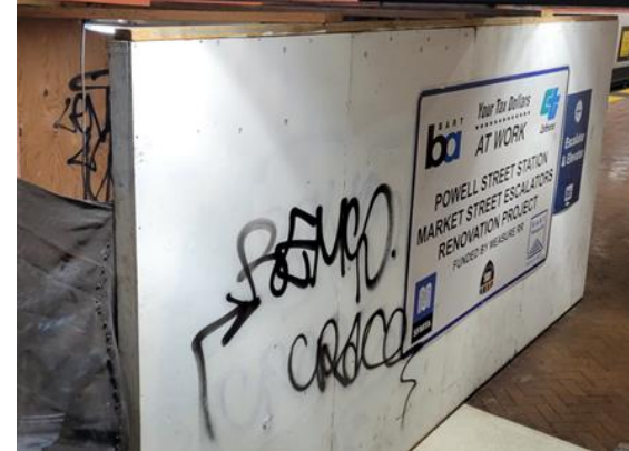
Vandalism, Property Theft & Bio-hazards Street Entrance of Civic Center Station
