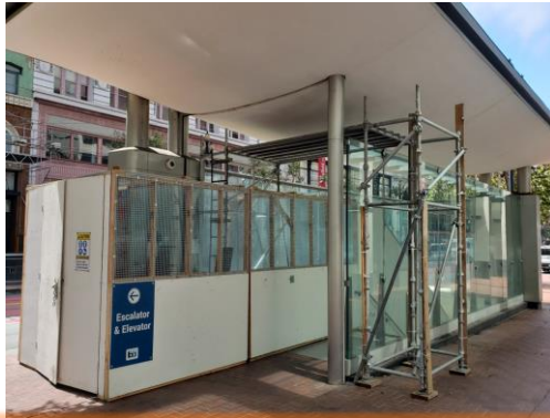
Project Schedule & Sequencing Escalator Construction after Canopy Completion
