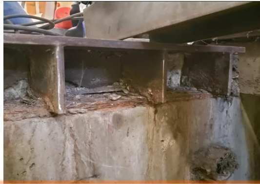
Differing Site Conditions Existing Escalator Truss Supports and Utilities
