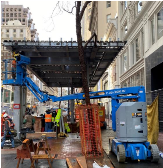
Metal Deck Installation
