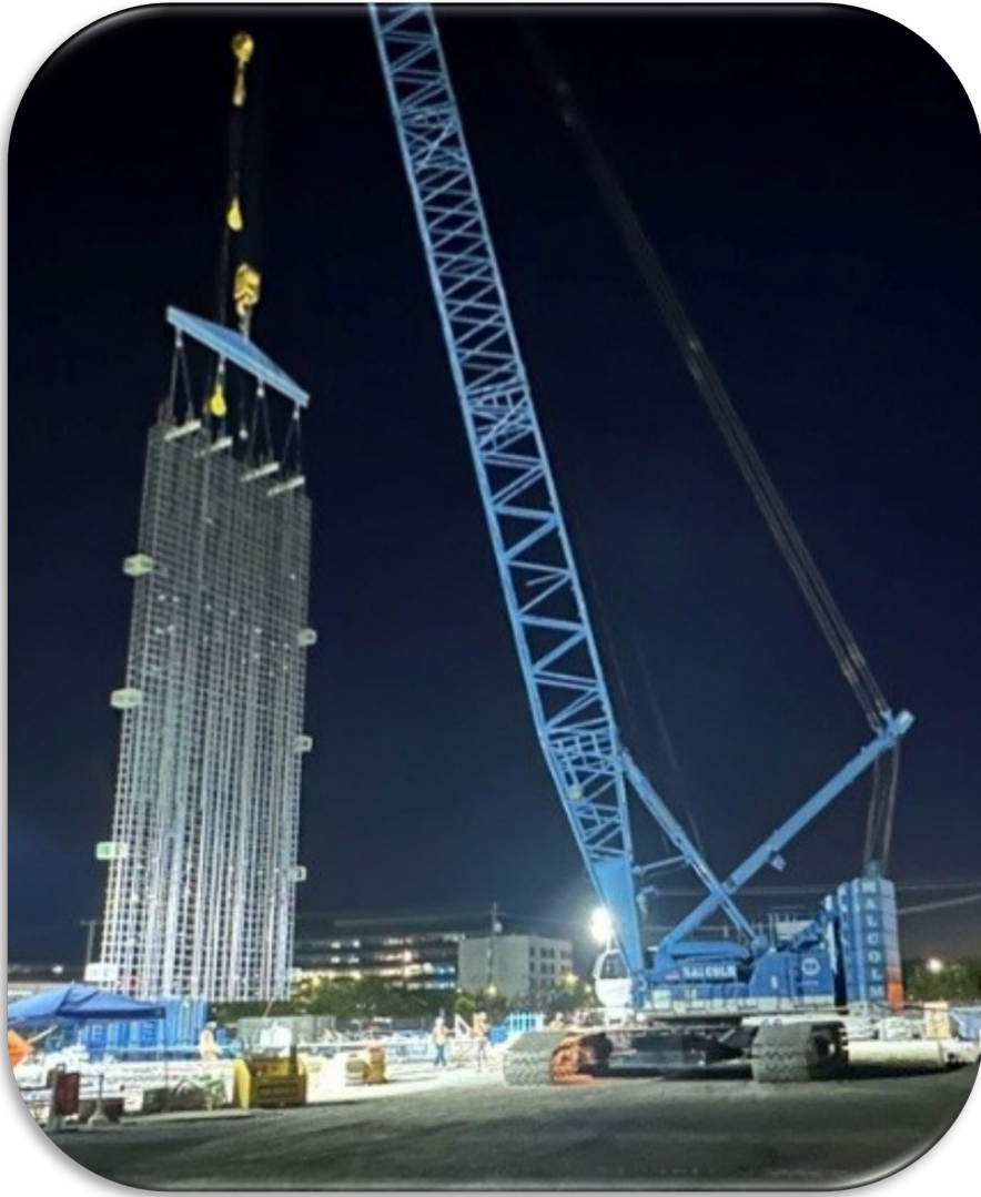
Placement of Rebar Cage for Structural Support Wall
