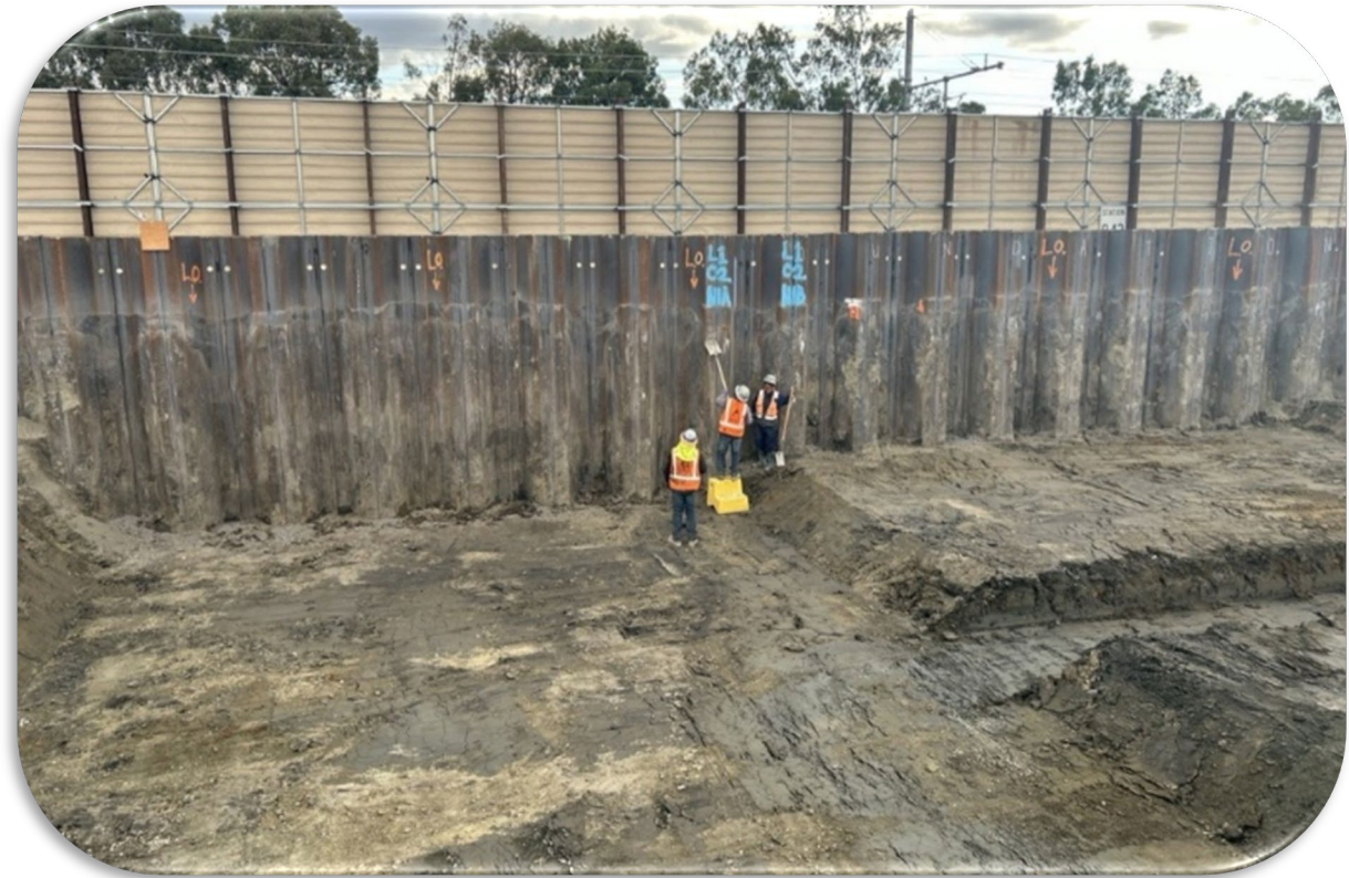
Mass Excavation Progress within Sheet Pile Area
