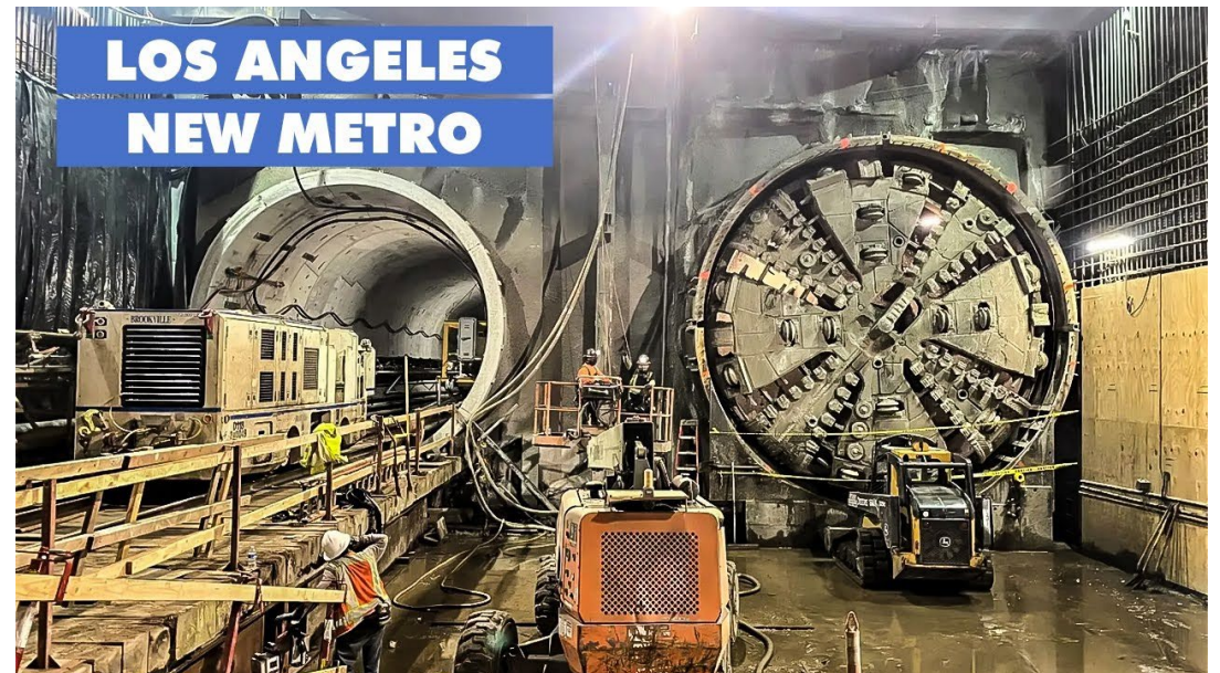
LA Metro's Purple Line TBMs
