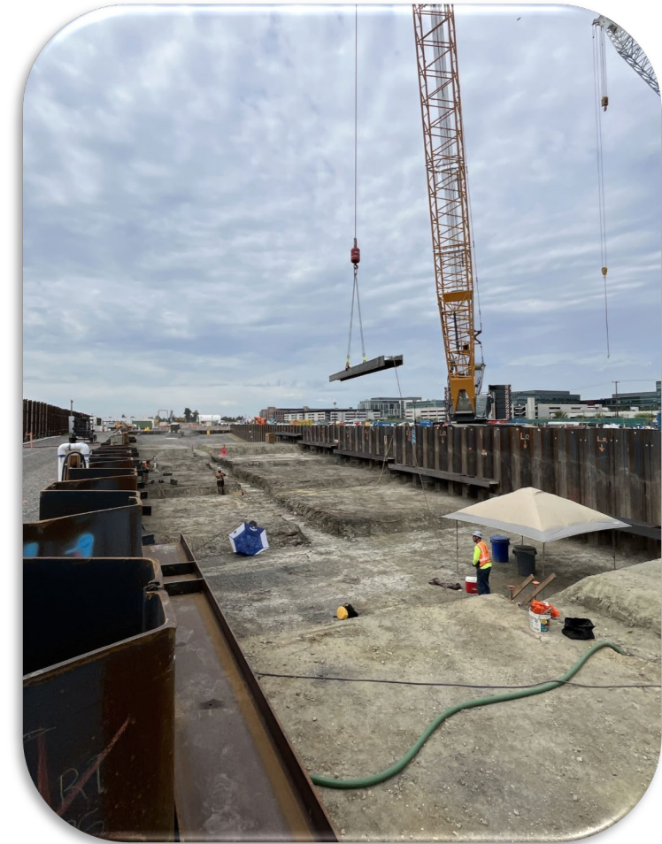
Ongoing Welding of Bracing Elements on the Sheet Pile Wall
