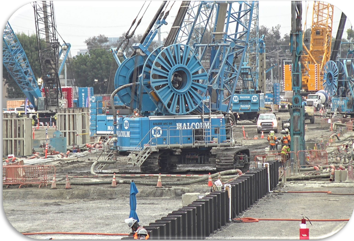
Ongoing Operations at West Portal Site
