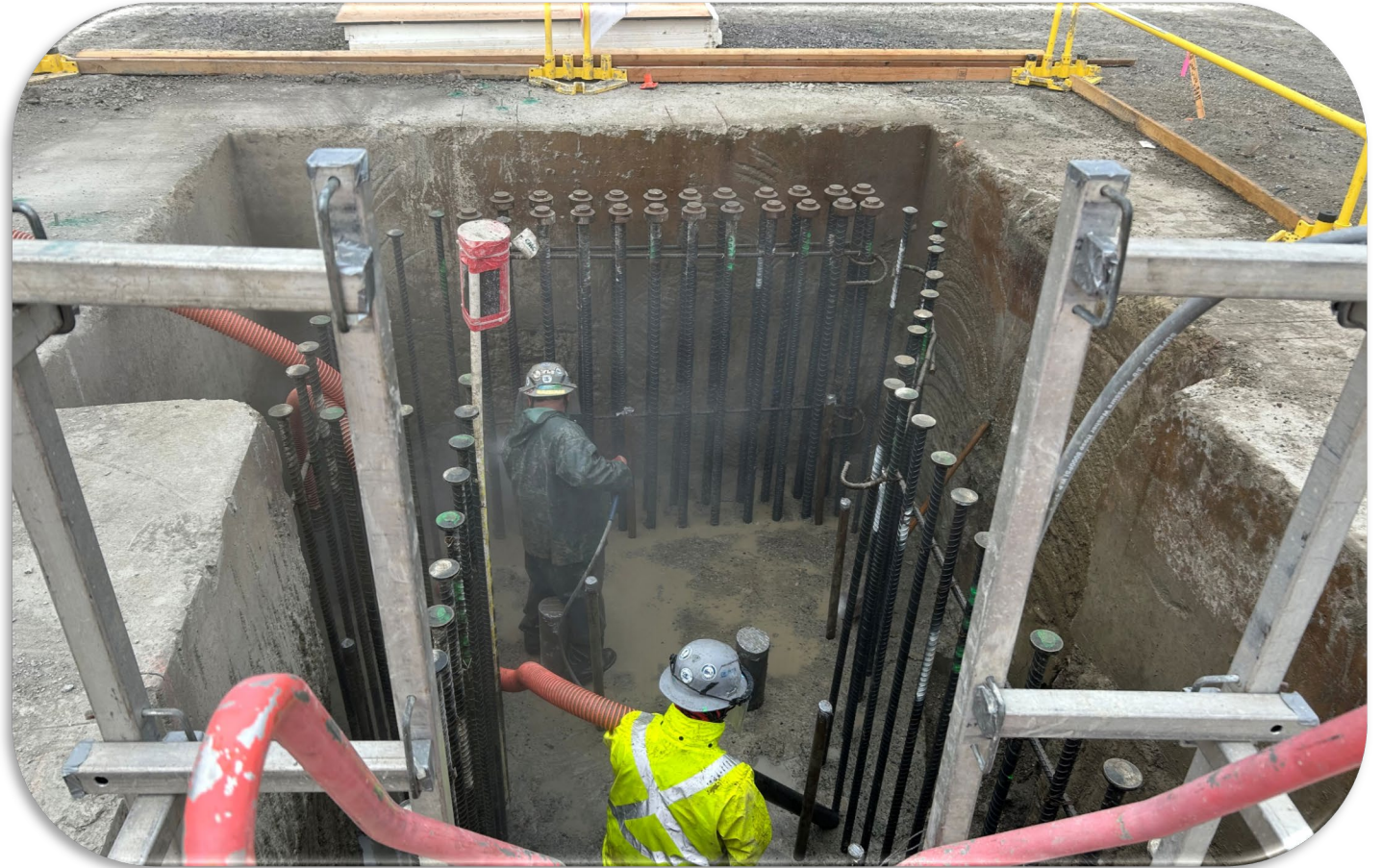
Pressure Washing of Y-Panel
