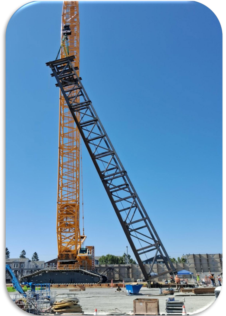
Crane Performs Lift Test for Rebar Cage Tripping Frame
