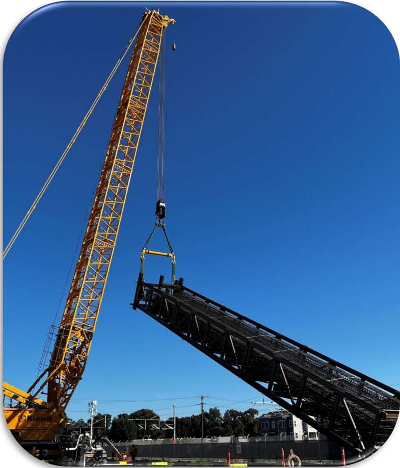
Crane Lift of Tripping Frame with the Y-Panel Rebar Cage inside
