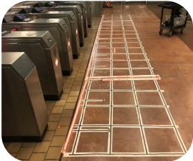
Built-in Conduits & Steel Bars
