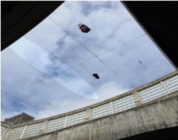
3 Safety Netting Replacement
