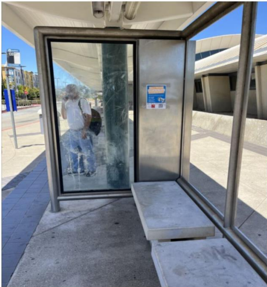
Bus Shelter Removal
