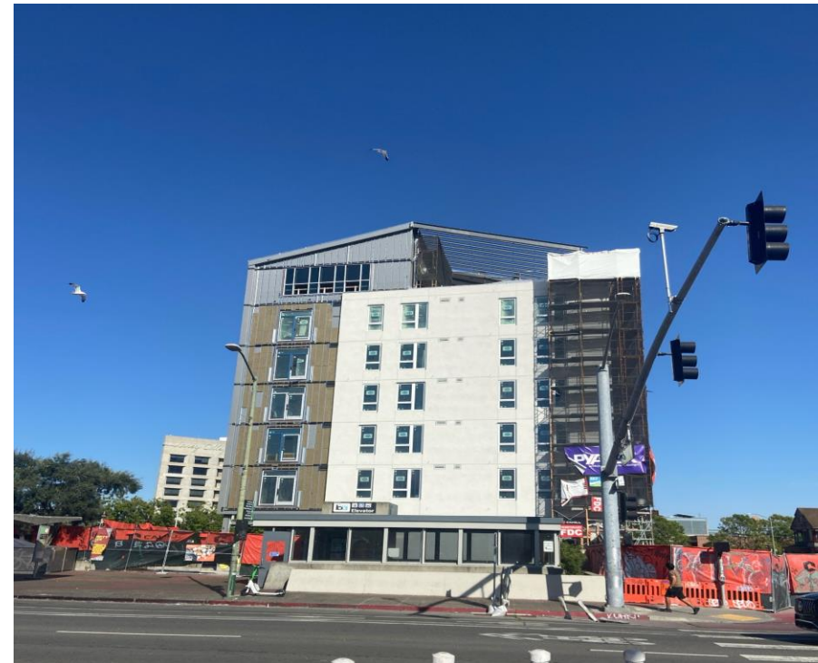
Clara E Chan Chinatown TOD in construction; Courtesy of EBALDC
