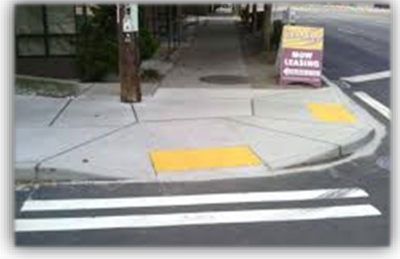
Accessible curb ramps
