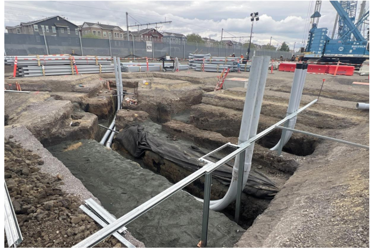
Medium Voltage Substation Conduit Excavation and Installation
