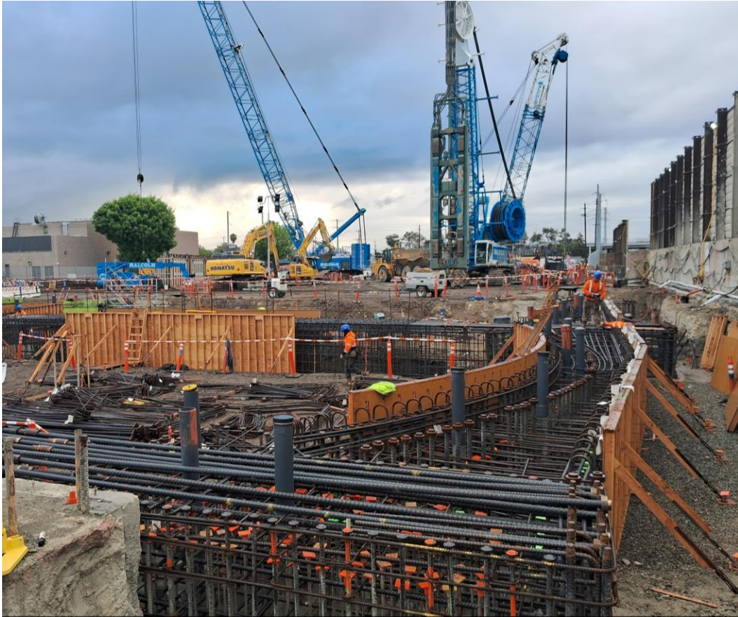
Caterpillar Shaft Cap Beam Rebar and Formwork Operations
