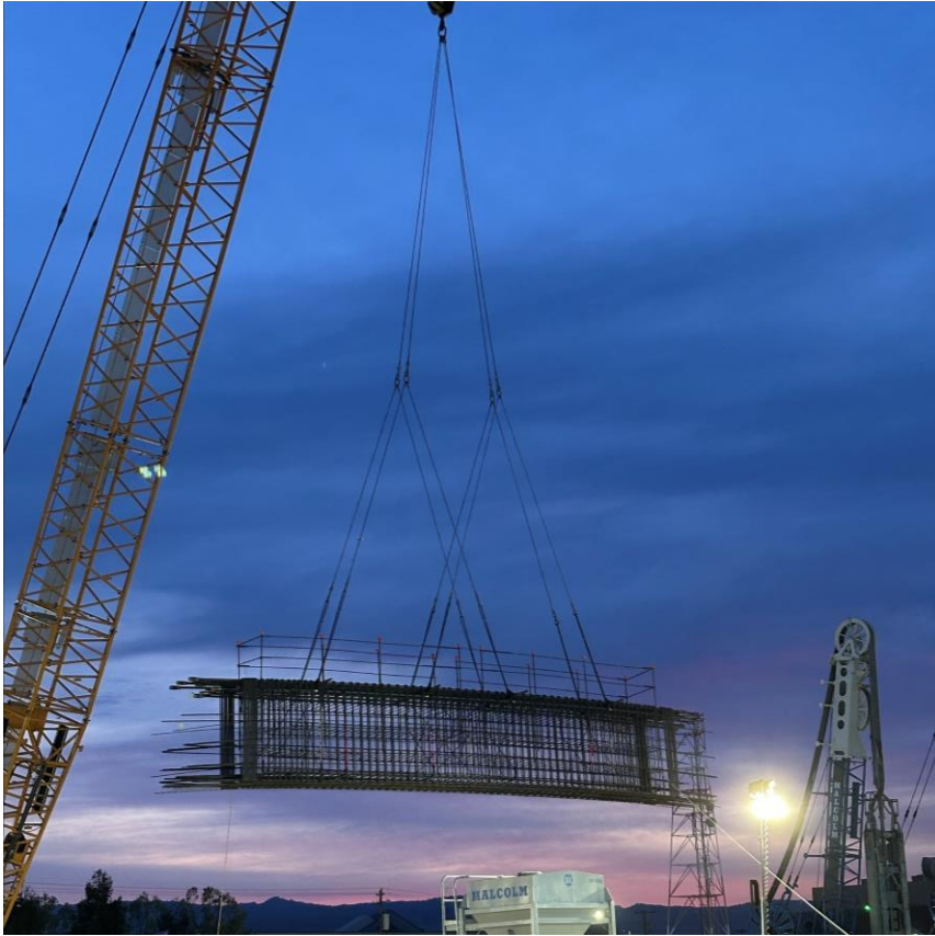
Caterpillar Shaft Top Strut Rebar Cage Lifting Operation
