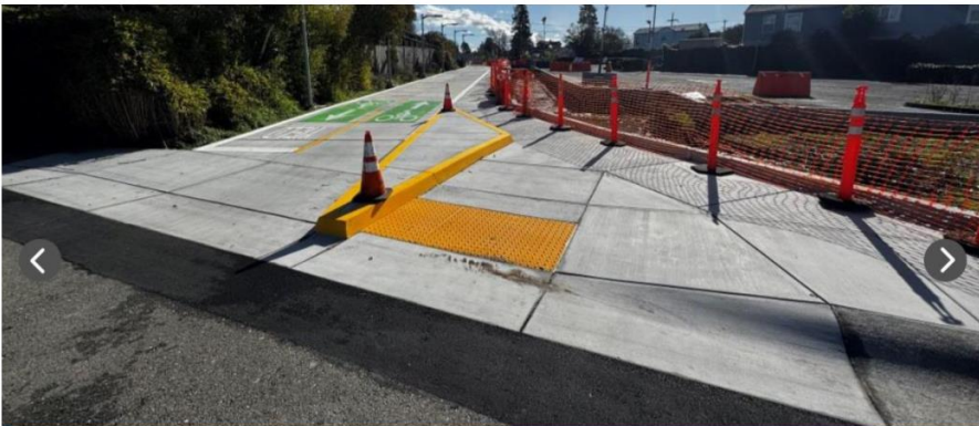
Widening of the Ohlone Greenway between the Acton Street/Virginia Street intersection and Virginia
