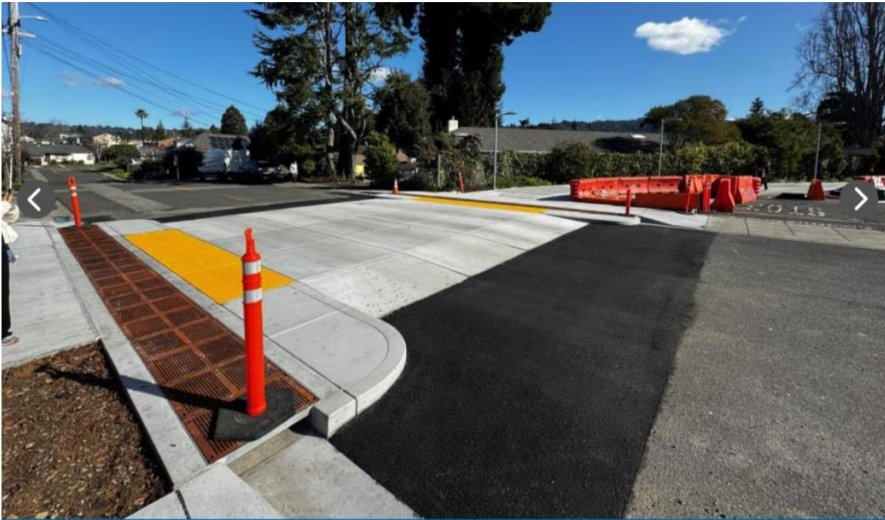
New raised crosswalk on Franklin Street at the Ohlone Greenway
