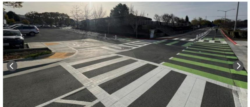
New separated two-way cycle-track on the BART access road between Acton Street and the station entrance and conversion to one-way northbound operation for vehicles
