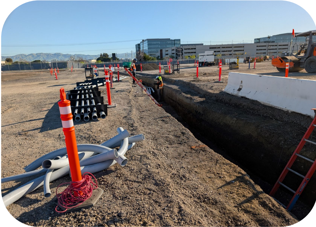
Trench and electrical conduit installation works
