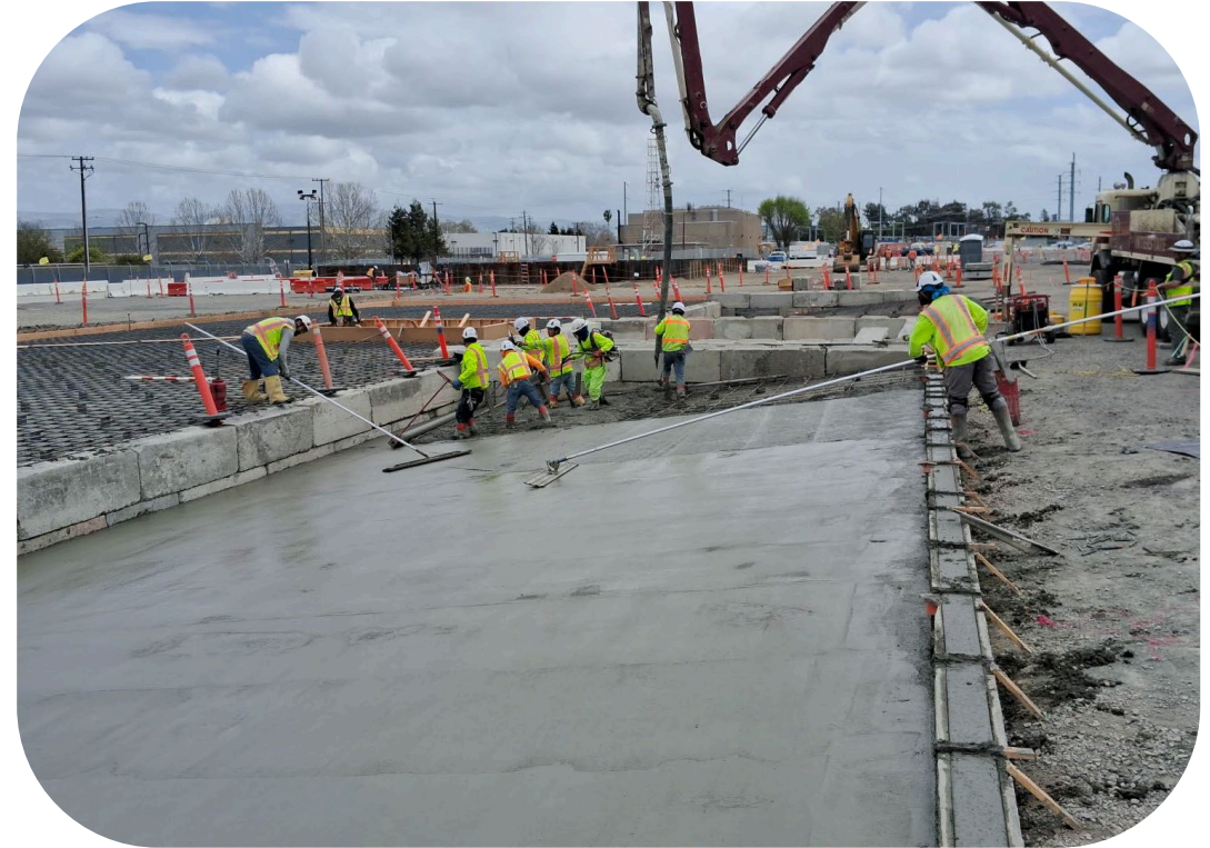
Concrete pour for the excavated materials bin
