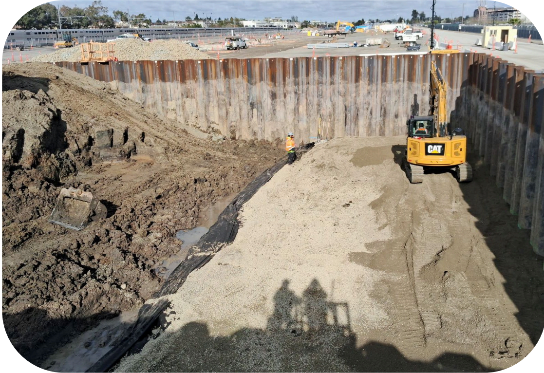
Excavation of detention basin
