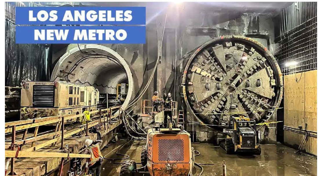
LA Metro's Purple Line TBMs
