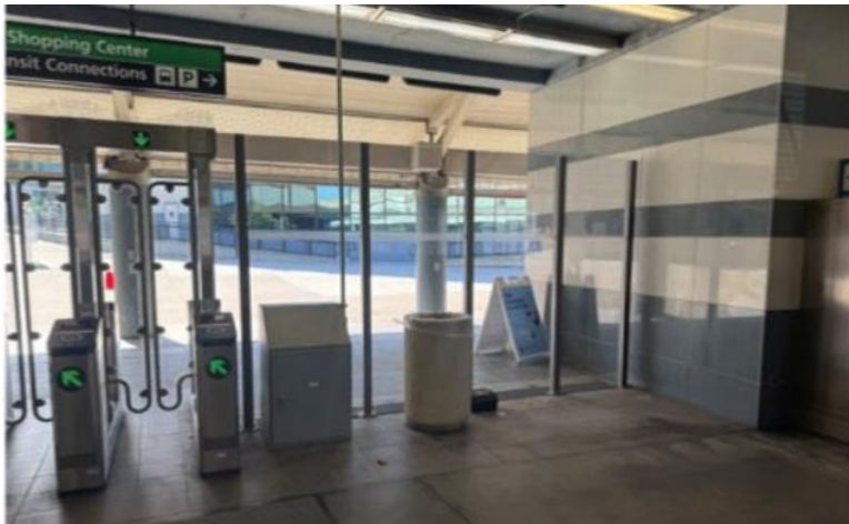
Lexan Barrier on New Steel Posts (San Bruno)
