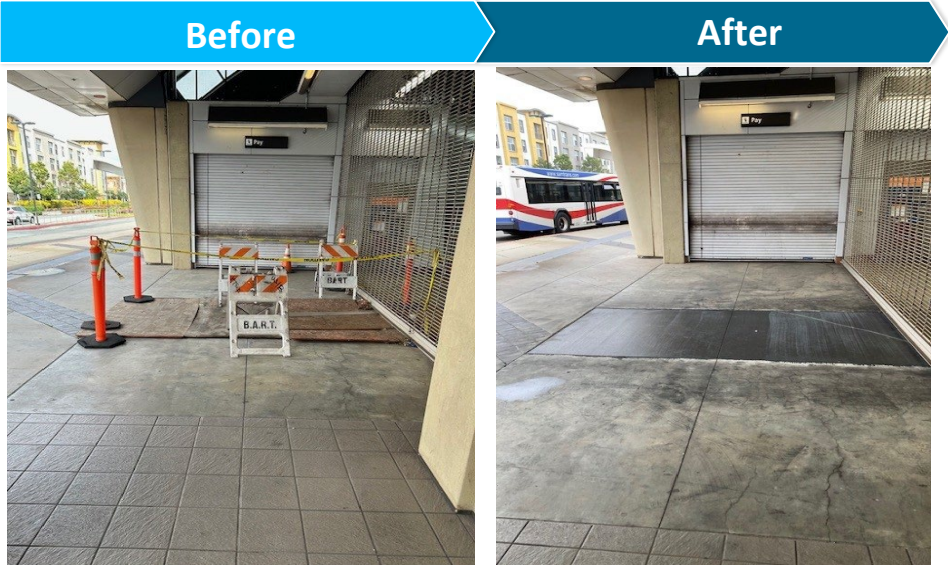
South San Francisco: Repaved Uneven Concrete Pavement
