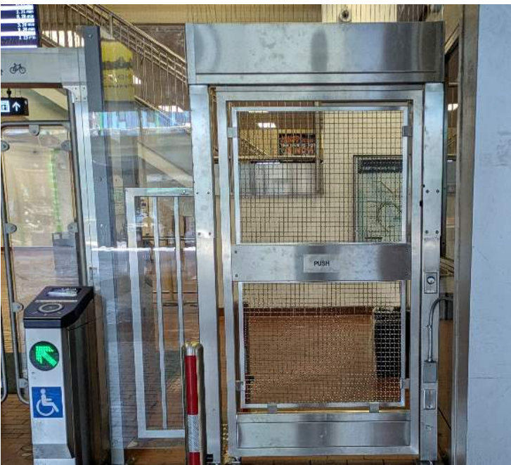
Mock-up of Swing Gate Installed on May 20, 2026
