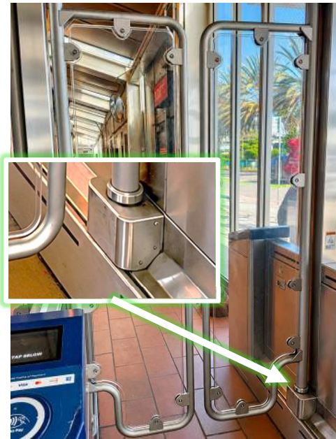
Detachable D Shaped Inserts Improve Maintainability without full Faregate Replacement or Repair
