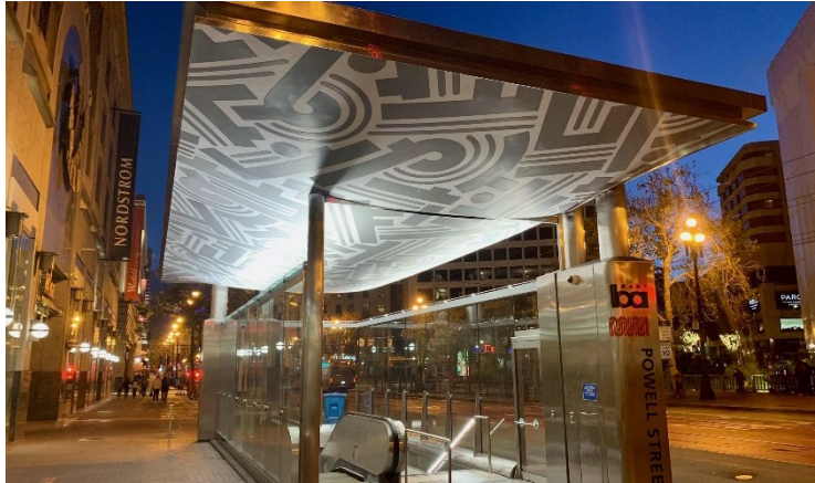
Market Street Entry Canopies
