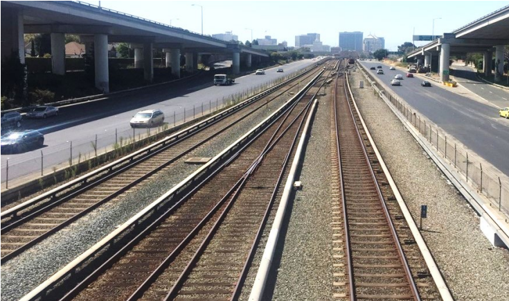
● Interlocking Replacement at Oakland Wye (K23 & K25)
