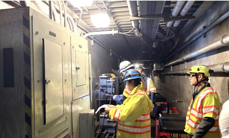
Traction Power Substation Installation (KTE)
