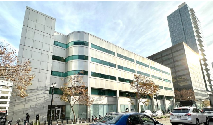
● BART Police Department Headquarters (BPD HQ)
