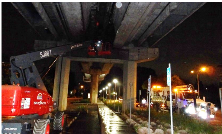
Traction Power & Train Control Communication (San Leandro)
