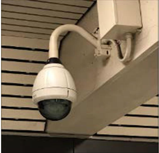
Sample Image of Semi-Visible CCTV Camera
